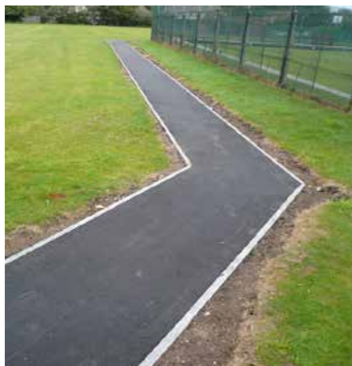
Asphalt Paths within open spaces
