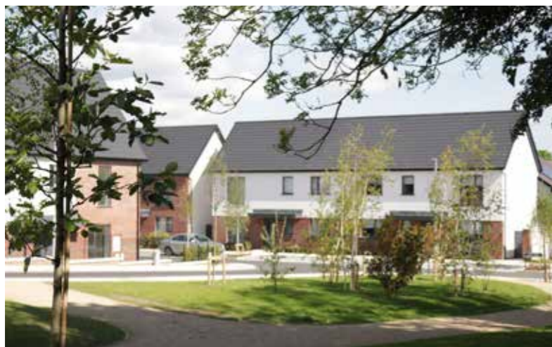
Site Photo from Newcastle Phase1 Open Spaces
