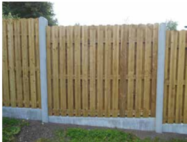
Timber Panel & Concrete Post: +1.8m to 2.0m - Within residential unit rear gardens
