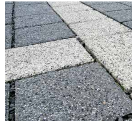
Permeable concrete block pavers used for driveways
